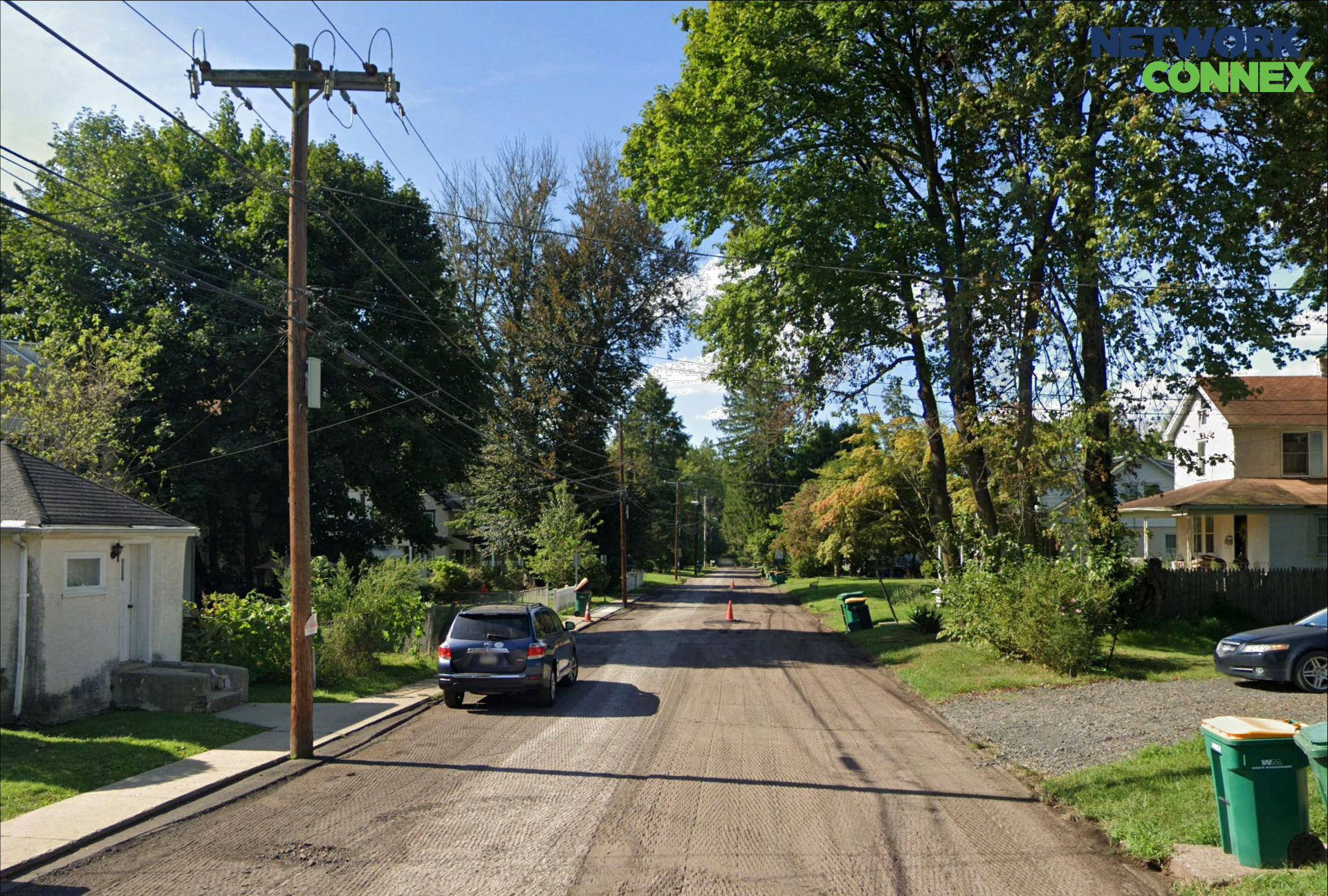
SITE NAME: LOWER GWYNEDD - PENLLYN WOODS PARK (RISE UP) VIEW 4 - 1100 TREWELLYN AVENUE EXISTING CONDITIONS
